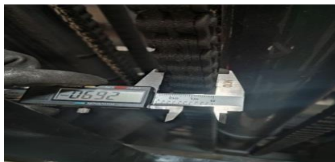
Figure 1. Forklift chain-thickness measurement.
