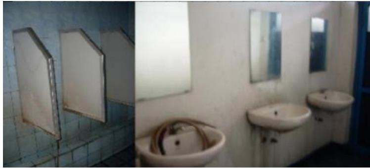
Gambar 1. Toilet Terminal Bus Giwangan, Yogyakarta
