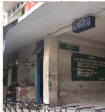
Gambar 5. Toilet Terminal Bus Giwangan, Yogyakarta
