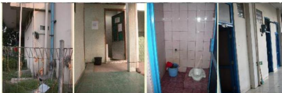
Gambar 3. Toilet Terminal Bus Giwangan, Yogyakarta
