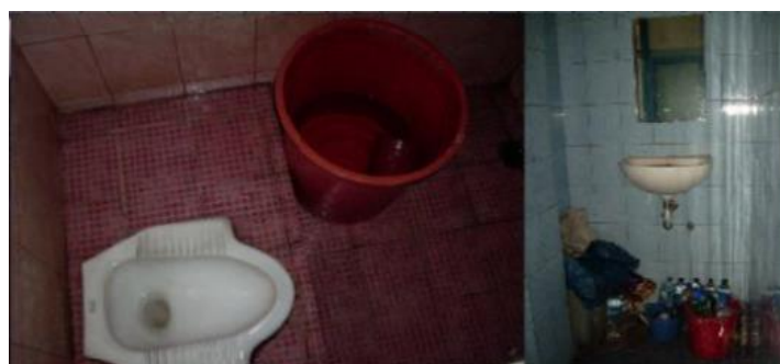
Gambar 8. Toilet Terminal Bus Giwangan, Yogyakarta
