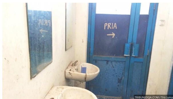
Gambar 7. Toilet Terminal Bus Giwangan, Yogyakarta
