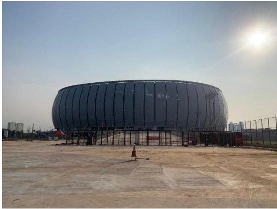
Gambar 1. Lokasi Penelitian di Jakarta International Stadium
