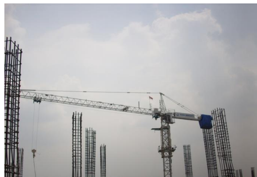
Gambar 2. Tower Crane merk Topkit FO/23B
